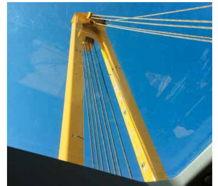
View to the boom through skylight in the cab roof
